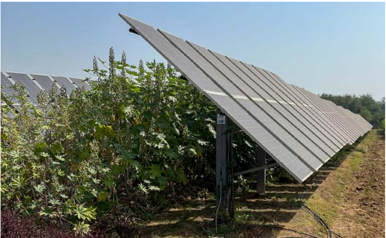
Agrivoltaics utilizes solar panels to use the same land to generate electricity and grow crops. (Photo by Milorad Plavsic/TCI)
